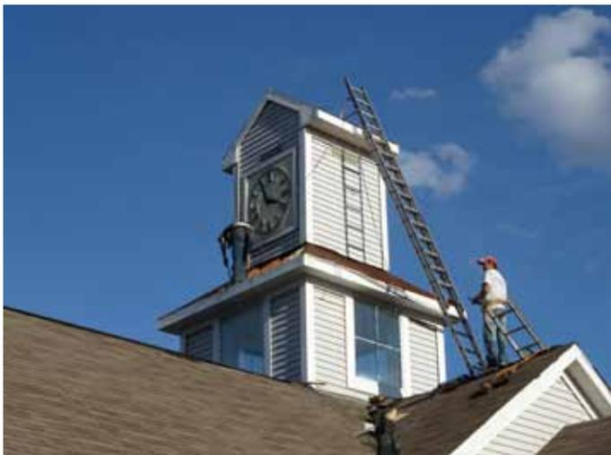
On Wednesday, February 22, while the monthly residents Council meeting was taking place, workmen descended upon the Clocktower and tore the roof apart. They removed the asphalt shingles from part of it, replaced rotting timber and sheathing under it and installed new roofing as needed. Back on Thursday, to finish the job, Ria Hawkins caught on camera the men working
